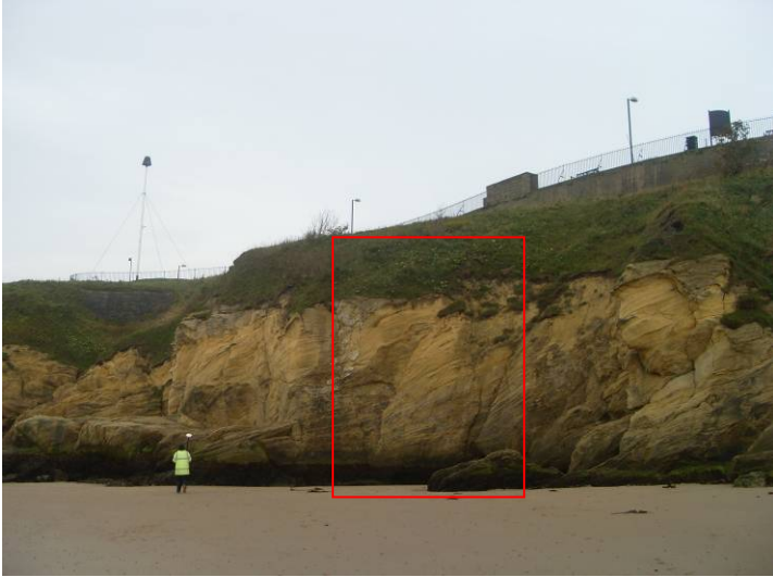
Plate 2 – Survey photograph, cliff face at profile 1aNTDC05 (1aNTDC05_20111027_S1.JPG)
